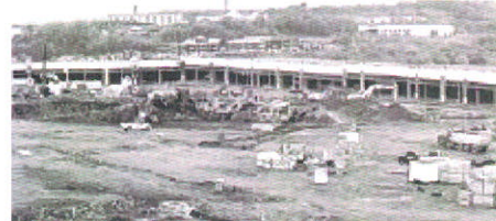
Construction continues on The Shoppes at Montage.
